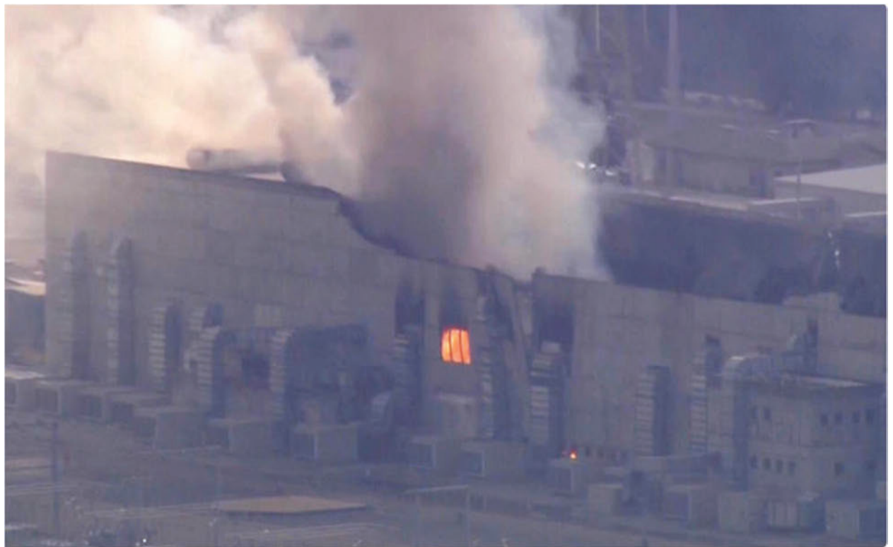
9 Figure 5 – Moss Landing Lithium Battery Facility Fire 7
