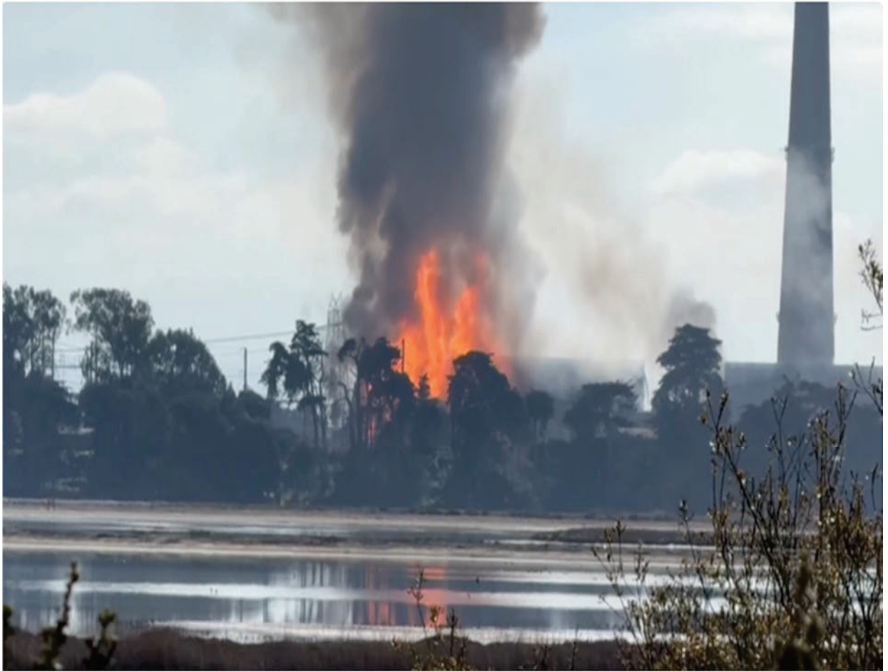
Figure 3 – Moss Landing Lithium Battery Facility Fire 5
