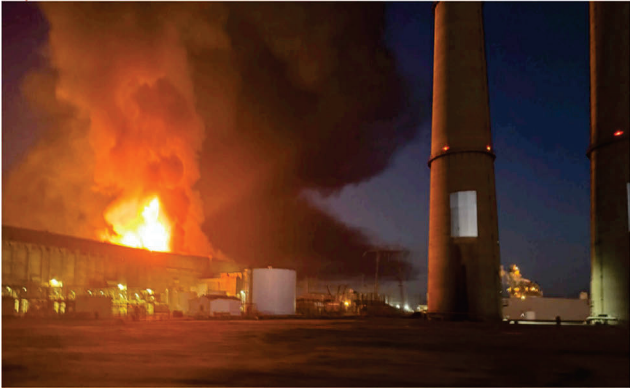
1 Figure 4 – Moss Landing Lithium Battery Facility Fire 6
